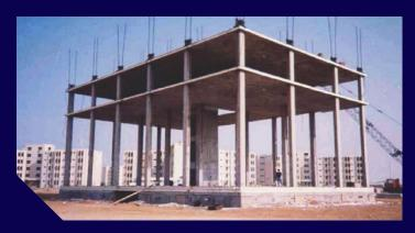
• First the columns are poured and then the jacking system is erected at the top of the columns, then the slabs are poured on the ground, lifted to its location and a cast in-situ part is poured to join the columns and the slab together.
