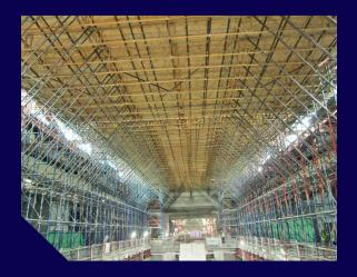
Acrow unit beams can be used with scaffolding tubes and couplers to build a full scaffold system that can make any required shape of scaffolds.
