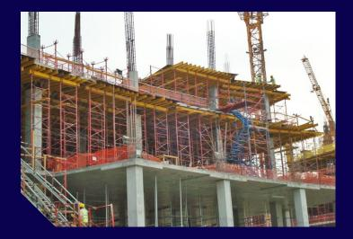
• The Shore-brace Table Form System is composed of standard components that can be used in different projects and different systems.
